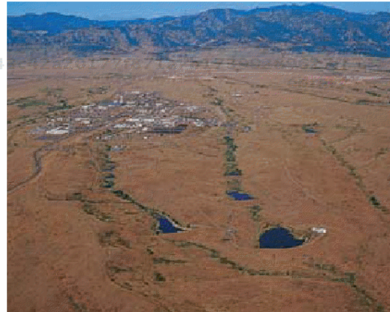
46—ASARCO Globe Plant Superfund Site, Globeville, Colorado, three miles north of Denver
